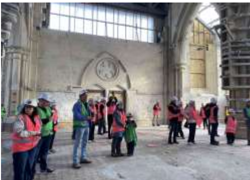
The view inside the partly repaired Christchurch Cathedral
